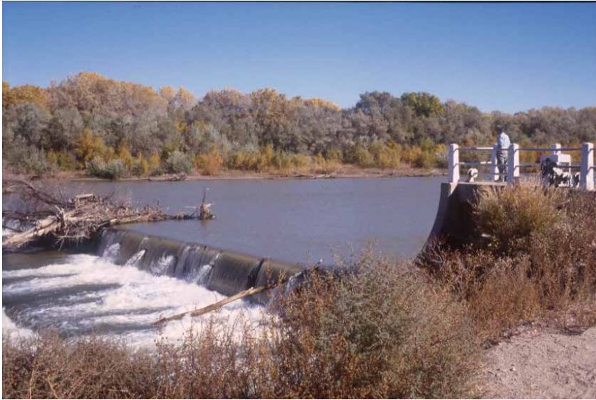
A diversion dam of the Middle Rio Grande Conservancy District near Algodones.
