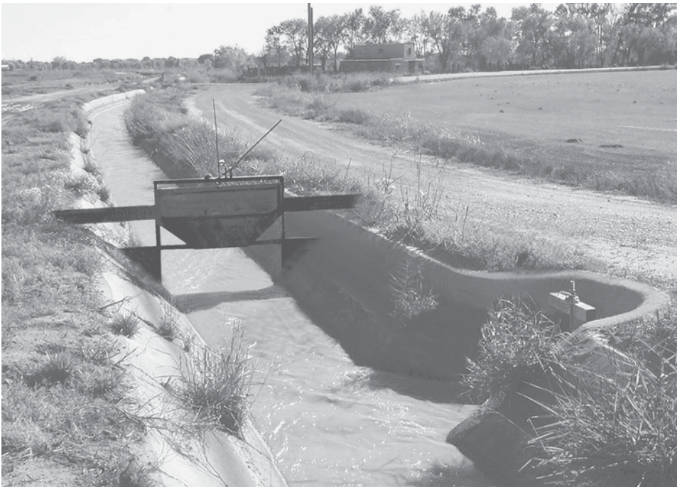
The metal structure on the left is a check. When it is closed the water in the high-line canal or lateral builds up to a level that will flow through the turnout, shown at lower right, into a farm field or smaller ditch.
